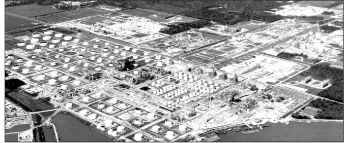
Security for Americas critical infrastructure requires proper planning by experienced professionals.
