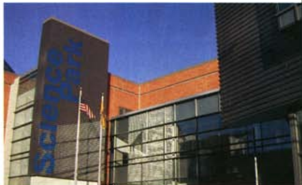
Newark Science Park High School, Newark, N.J. Photo courtesy of M. Michalski / Professional Systems Engineering, LLC
